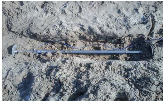
Model 4430 Vibrating Wire Deformation Meter installation.
