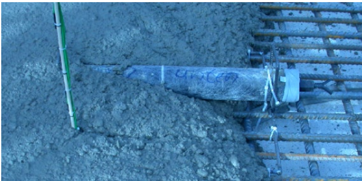
Figure 3 - Concrete being poured around the stressmeter
