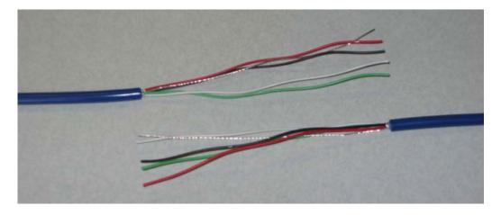
Cut conductors in staggered pattern and strip ends 3/8":
