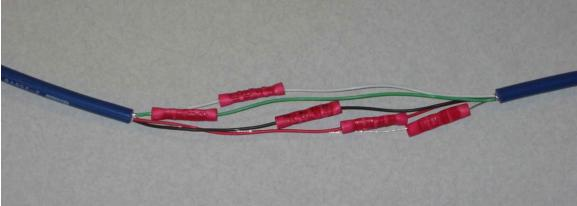
Gently twist cable and lay in one mold half, with splice area centered:
