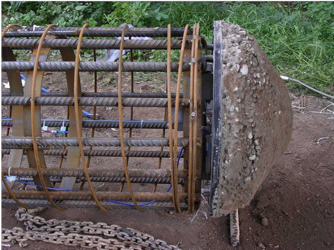
FIGURE 2: Pressure Cell (With Concrete Cone) Installed on the Rebar Cage
