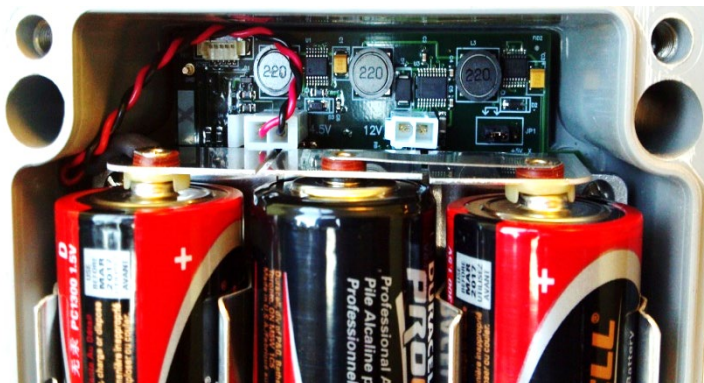
Figure 18 - Datalogger Battery Pack Connections
