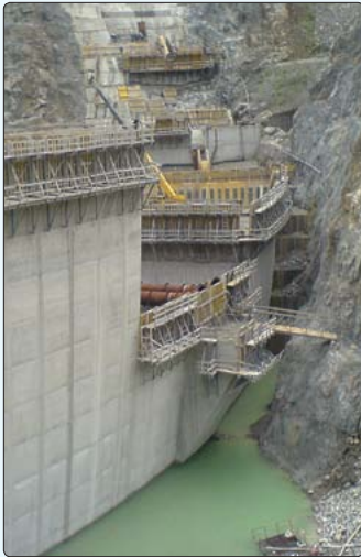
• Downstream view of right bank under construction.
