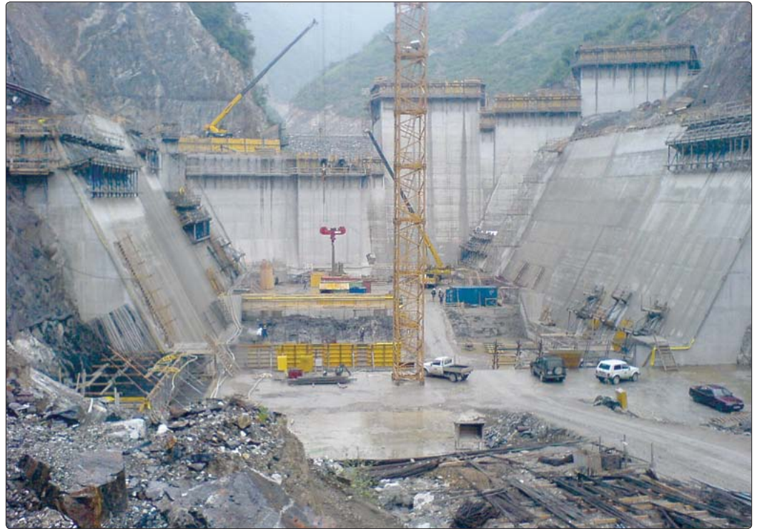
• The Tsankov Kamak Dam, Devin, Bulgaria.
