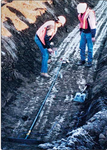
● Installation of Model 4435 sensors.
