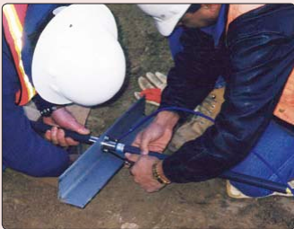
• Attaching the end flange.
