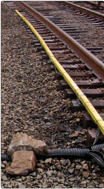
● MEMS Tilt Beam (fiberglass version) installation alongside railroad tracks.
