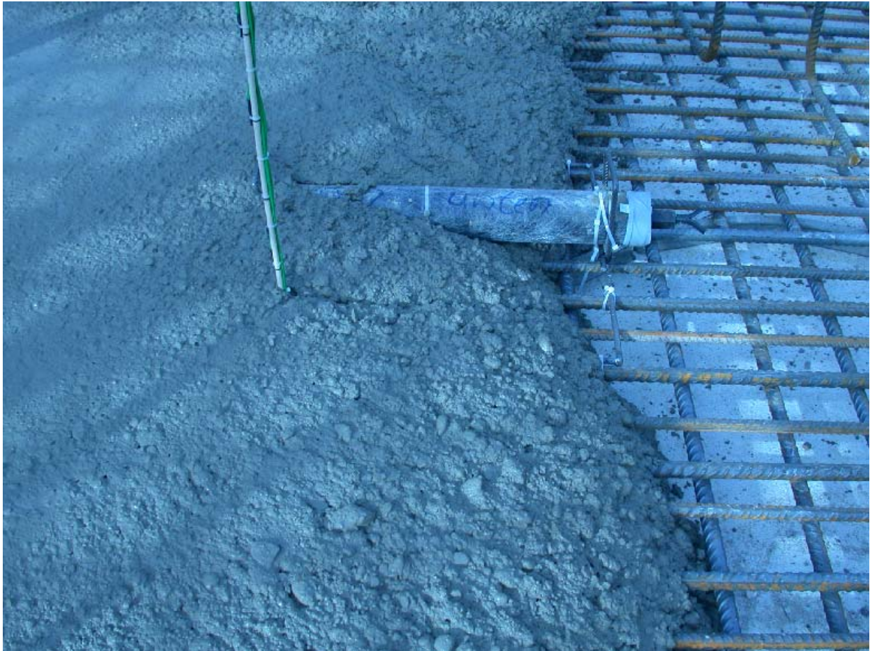
Figure 4. Concrete being poured around the stressmeter
