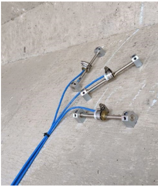
Vibrating wire strain gauge rosette installed on a girder's web
