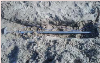
• Model 4430 Vibrating Wire Deformation Meter installation.
