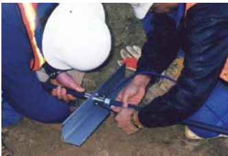
Attaching the end flange.
