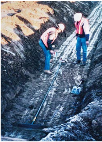
Installation of Model 4435 sensors.
