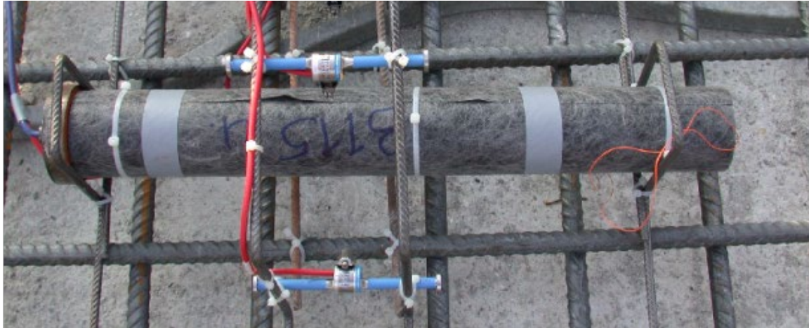
Figure 2 - Stressmeter ready for concrete pour
