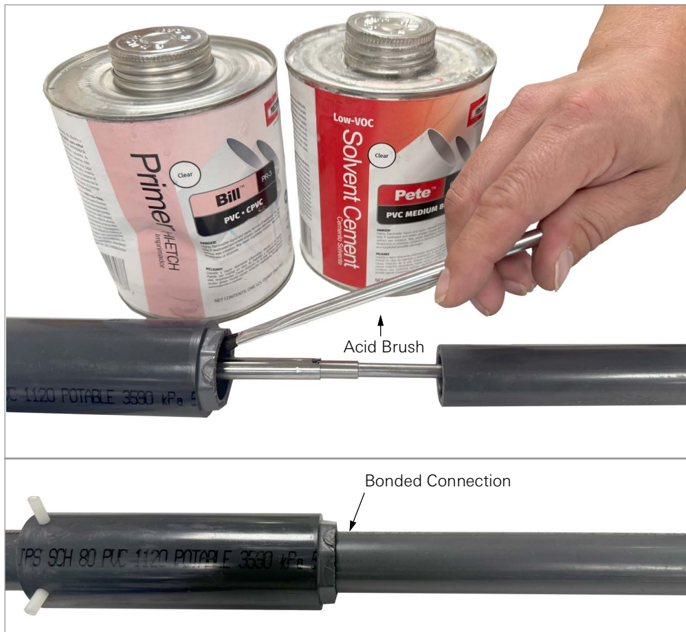
FIGURE 8: Install Pipe Onto the Receiving Adapter (Top), Completed Connection (Bottom)
