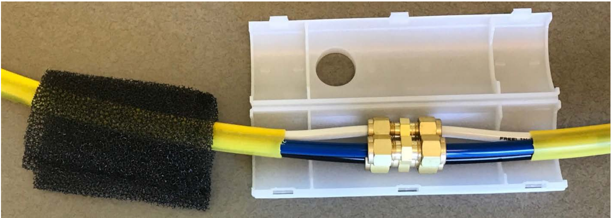
Figure 10 - Swagelok Fittings Installed
