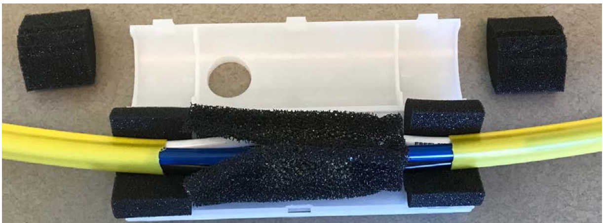
Figure 11 - Large Pieces of Foam Installed
