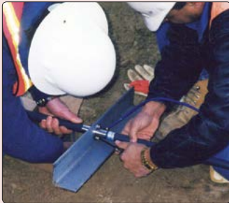
• Attaching the end flange.
